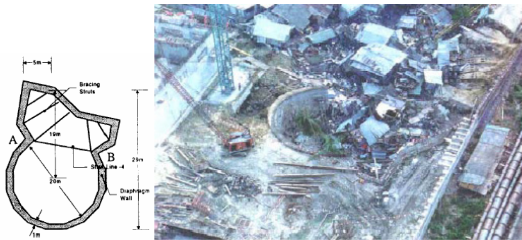
Figure 3. Collapse of an inlet pumping station (Teparaksa, 1999).
